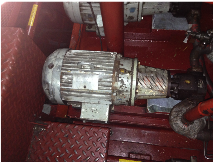
Figure 5. CPP "C" pump motor that supplies pressure to vary the pitch on the blades of the propeller. These pumps are energized when RMD is set and the vessel enters a time of increased risk and fatigue for the crew.
