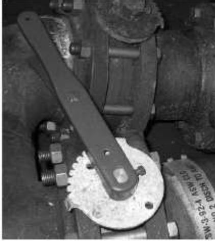
FIGURE 12: ASW throttling valve
