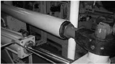
FIGURE 14: Rudder stock and tie rod
