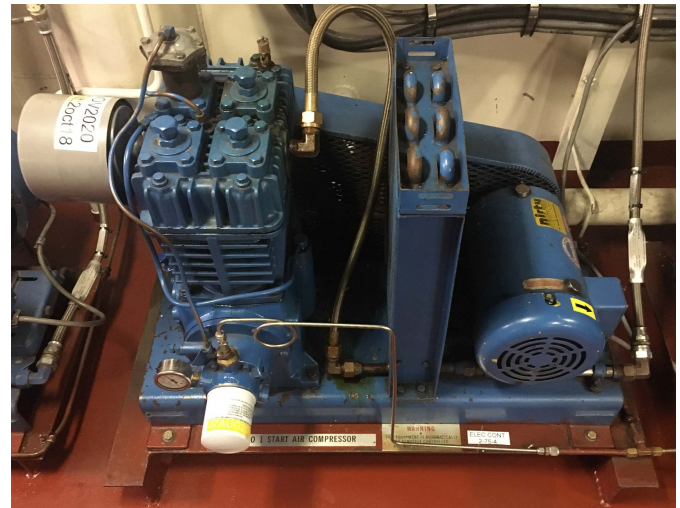
Fig. 18. Quincy QR-25 model number 325 two-stage compressor.
